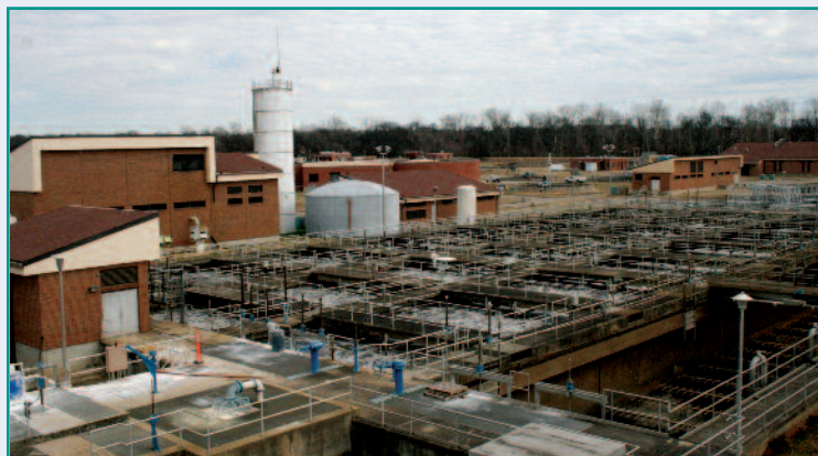
When rags and similar items are improperly disposed of within the MWA system, they can negatively impact sewer pumping equipment and operations at the Authority's lift stations and wastewater treatment facilities, such as the Lower Poplar Plant (above).
