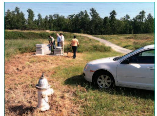
**A crew from the MWA and Cavanaugh & Associates performs a field inspection of an existing bulk customer meter, to verify meter condition and configuration of piping connections.**
