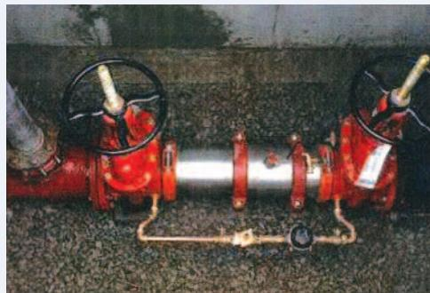
**This backflow prevention device, which is installed on the customer's side of the water meter, protects MWA drinking water from contaminants that might enter the system from cross-connections to potential sources of pollution.**
