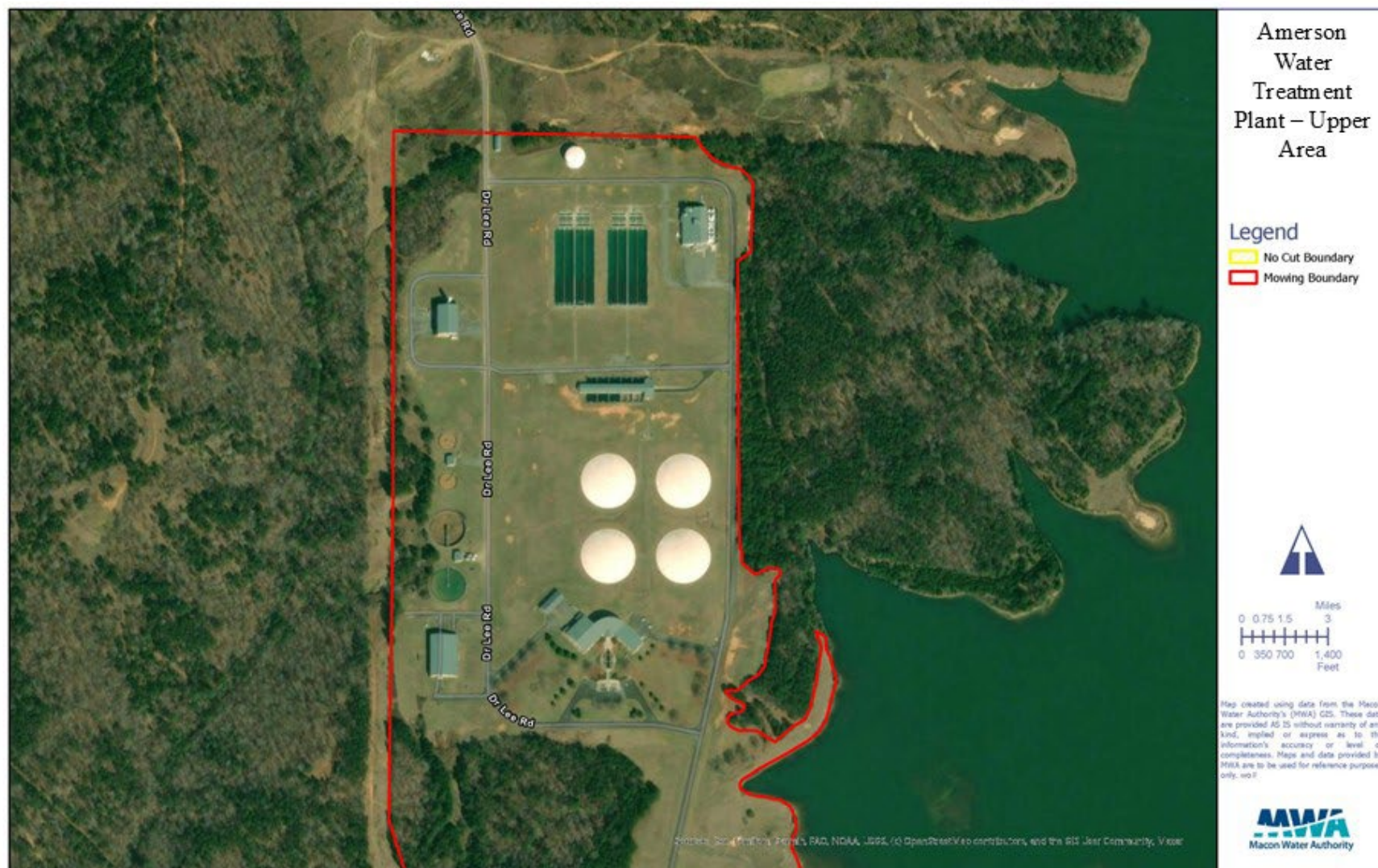
Exhibit "B" – Amerson Water Treatment Plant – Upper Area
