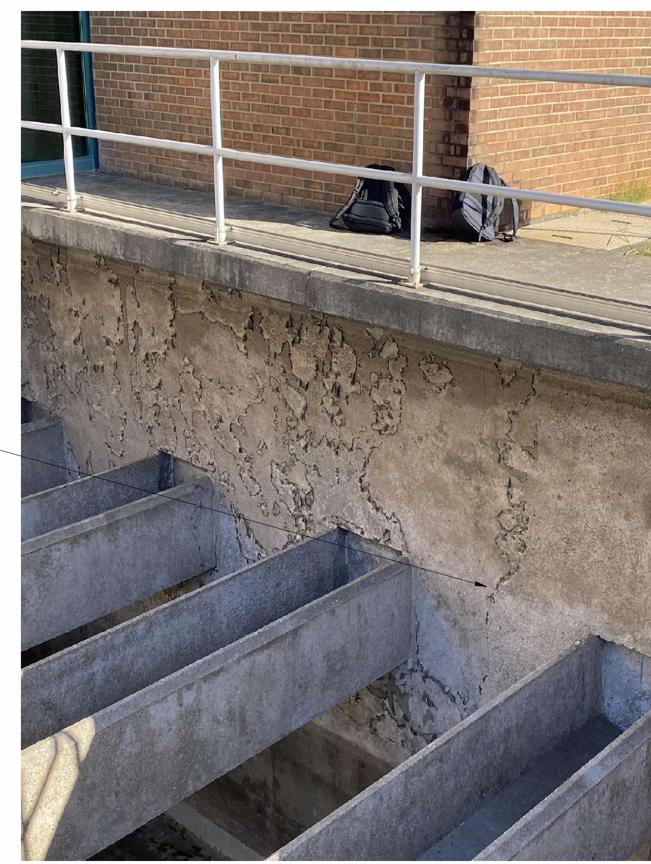
4 PHOTO #03 - FILTER PIT WALL REPAIR SB301 NTS
