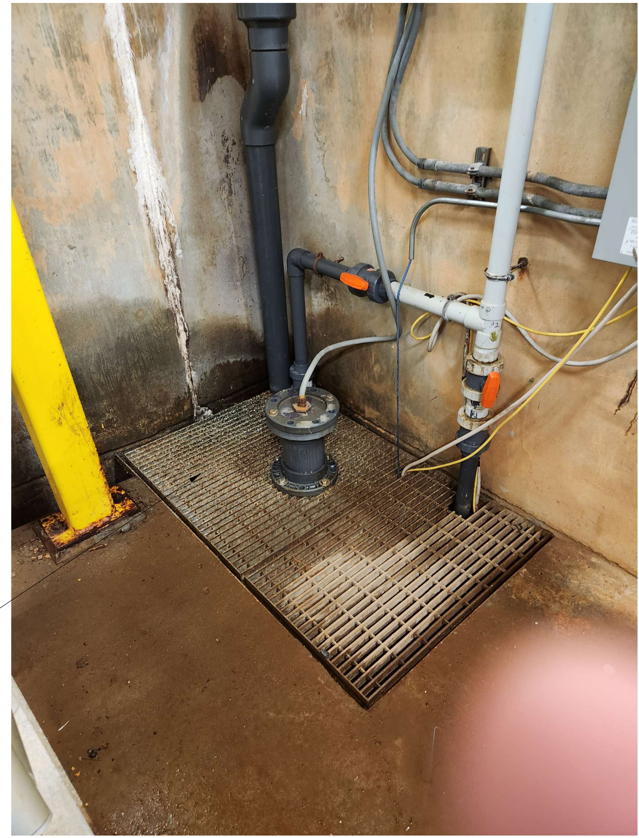
2 PHOTO #13 - STEEL PLATE AT SUMP PUMP PIT SB303 NTS
