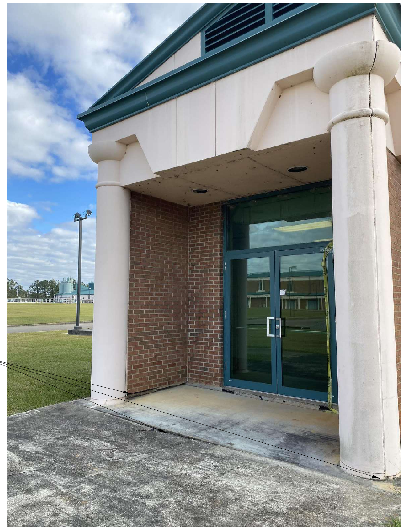
1 PHOTO #12 - WEST PORTICO SB303 NTS
