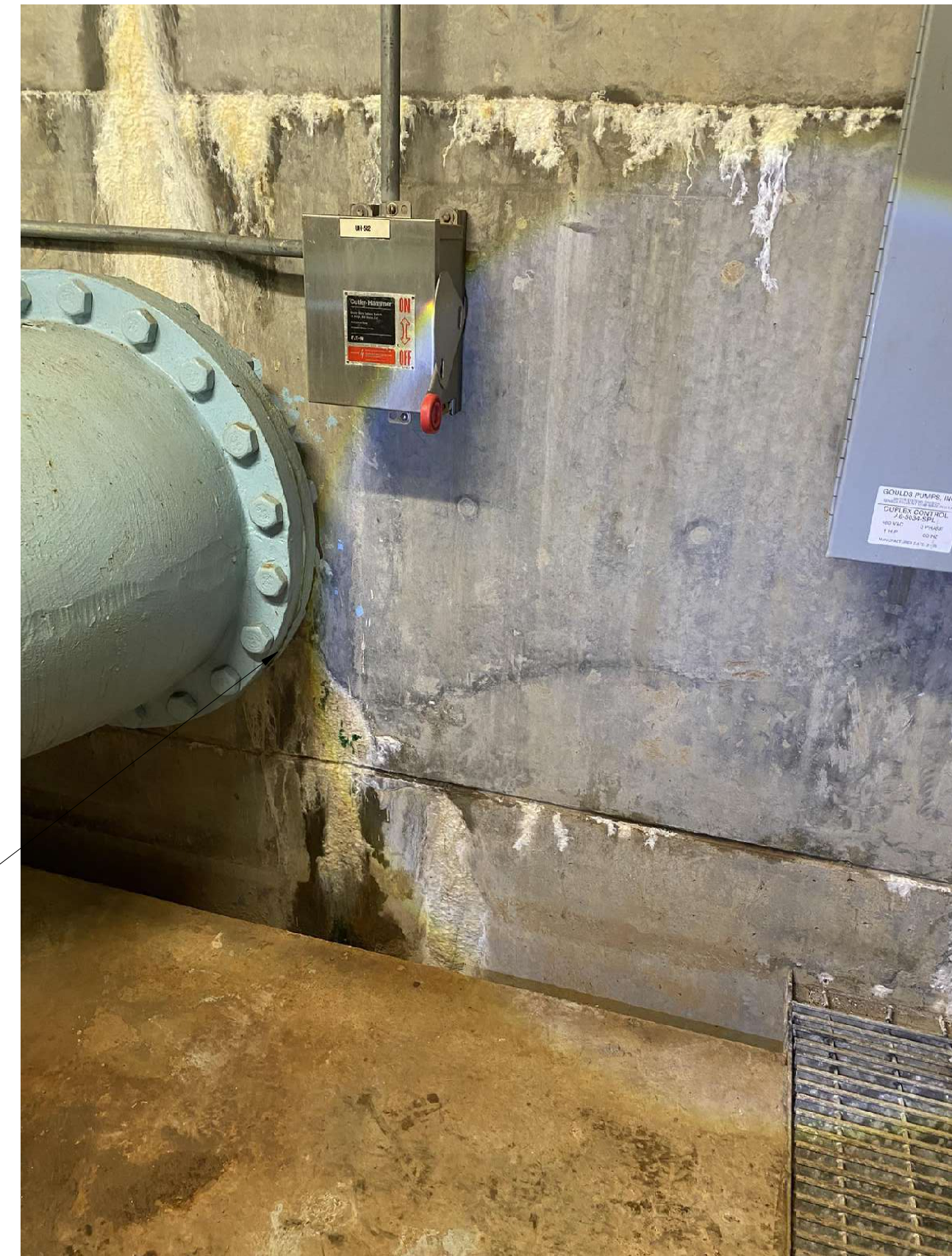
1 PHOTO #06 - PIPE PENETRATION SB302 NTS
