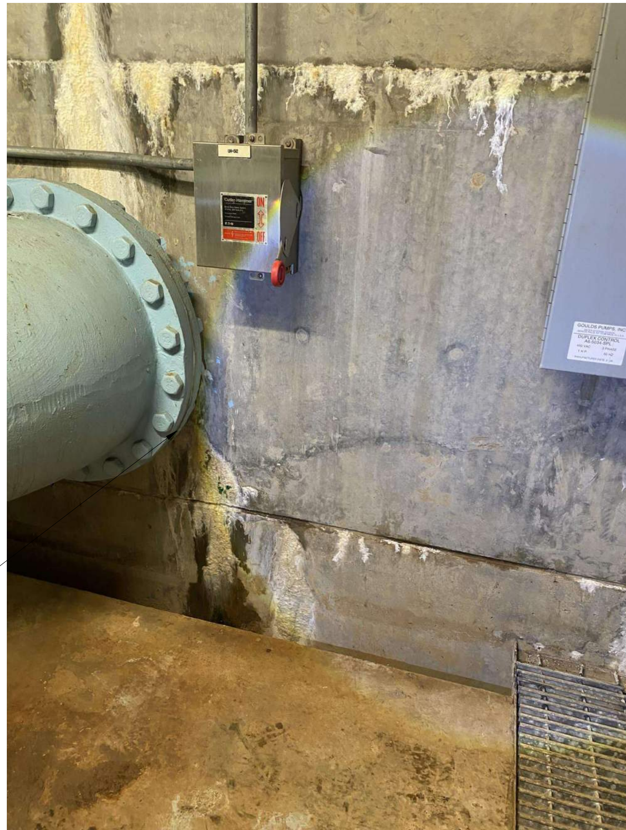
1 PHOTO #06 - PIPE PENETRATION SB302 NTS
