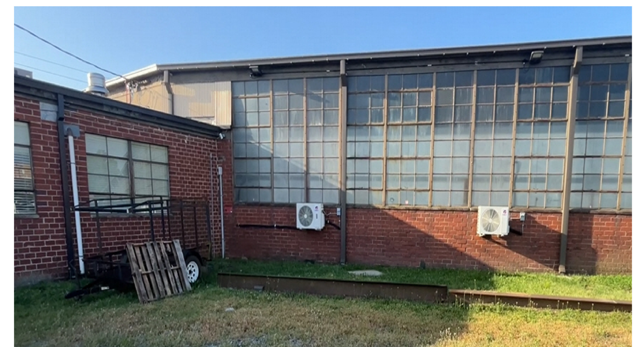
SOUTHWEST CORNER DETAIL
